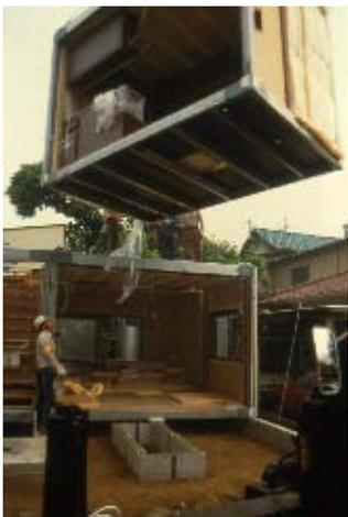
*Figure 8\*: Onsite assembly of a box unit house*
