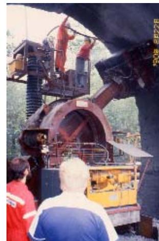
*Figure 9\*: Robotic concrete roller for tunnel construction*
