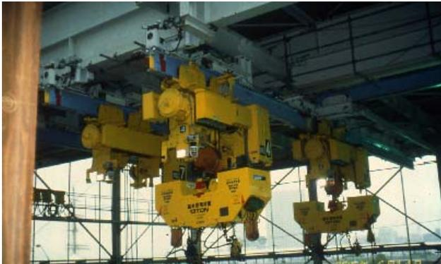
*Figure 16\*: Two of 22 robotic trolleys for transporting and positioning of beams, columns, floor panels, building services units and facades*
