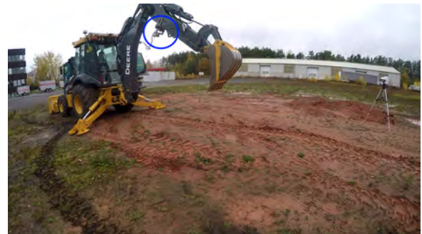
Figure 1. Excavator with additional sensor system (blue circle)
