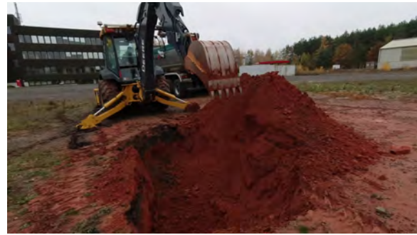
Figure 5. Final excavated trench
