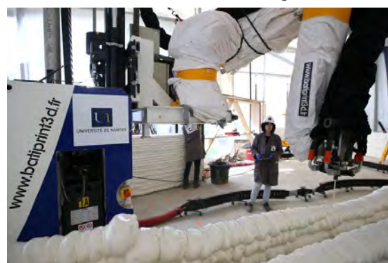
Figure 1. Additive foam manufacturing: BatiPrint3D, Yhnova's house 3D Printing with an AGV and a serial robot
