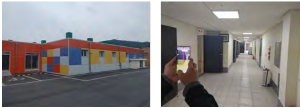
Figure 4. The outside and inside of the office building for test
