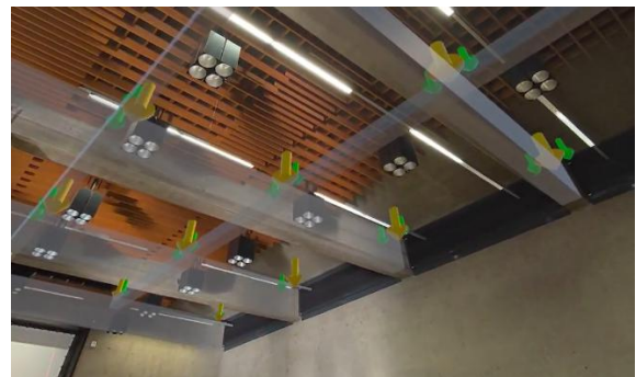
Fig. 3 Load transfer of a ceiling structure visualized in AR (overlay of the physical space), view facing the interior wall. [Own Illustration]
