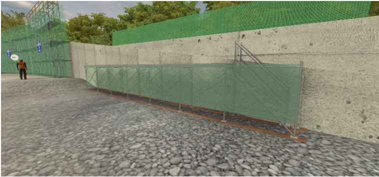
Fig. 2 Identifying Missing Safety Components
