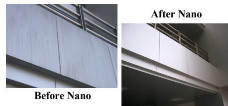
Figure 3. Out-wall before/after use Nano Coating.
