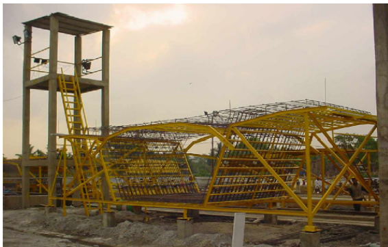
Figure 1. Reinforcement for Segment
