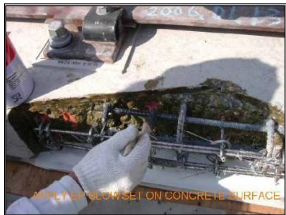
Figure 12. Reinforce and surface bonding layer
