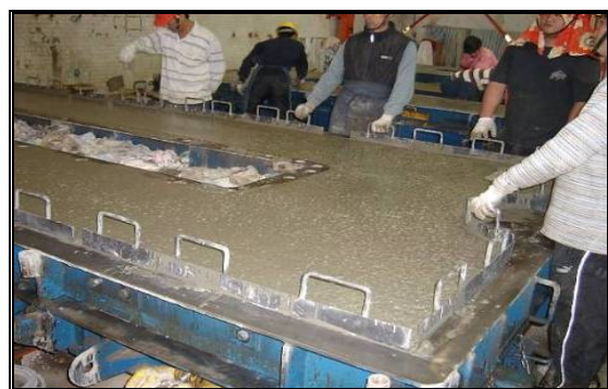
Figure 15. Steel plates used to extract bubbles
