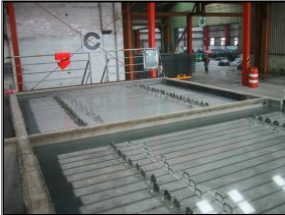
Figure 9. Curing of slab tracks in water
