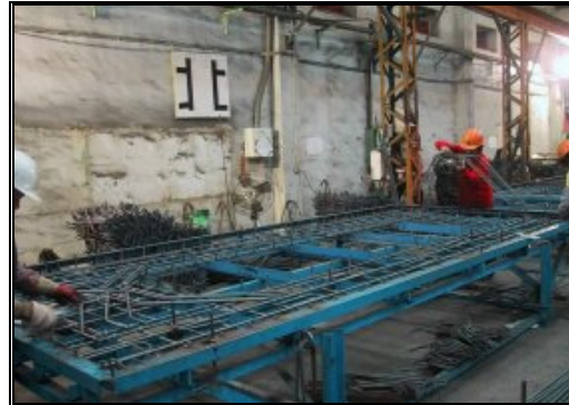
Figure 5. Assembly platform for reinforce cage
