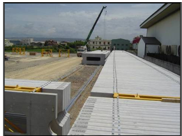
Figure 11. Slab storage area
