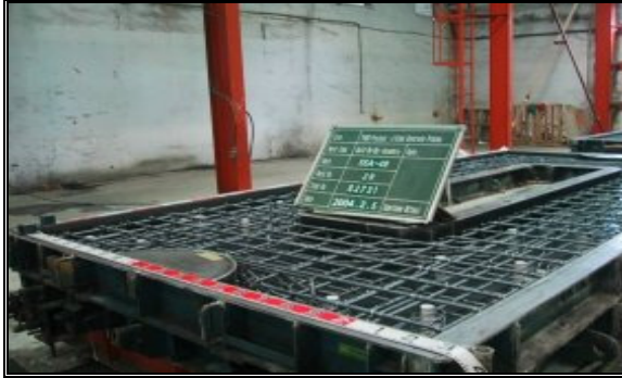
Figure 6. Inspection of reinforcement
