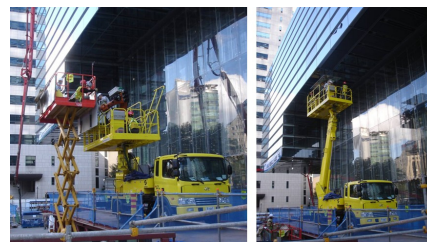
Figure 8. Loading & lifting of a glass ceiling
