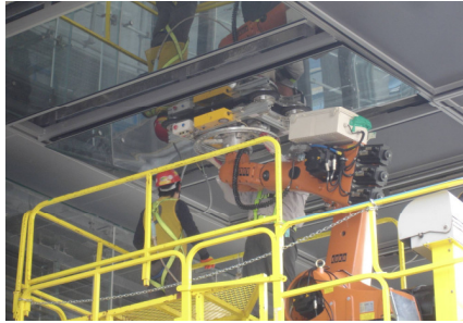
Figure 9. Installing & finishing of a glass ceiling
