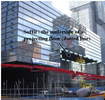
Figure 1. Construction site and soffit for building
