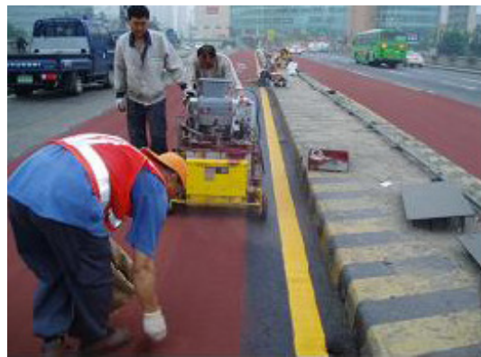
Figure 2. Melting-blown ultra-thin layer color pavement construction
