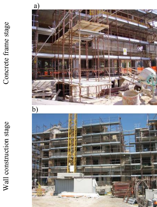
Figure 2. Two main stages of the construction site
