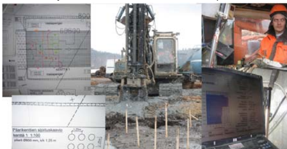
Fig. 1. Traditional process of deep stabilization.
