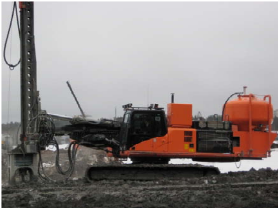
Fig. 7. A 3-D Controlled Deep Stabilization Machine.
