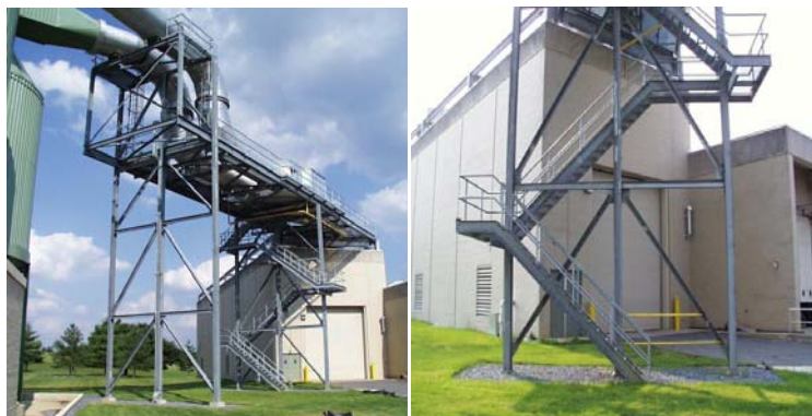
Figure 6: Steel Structure on NIST Main Campus
