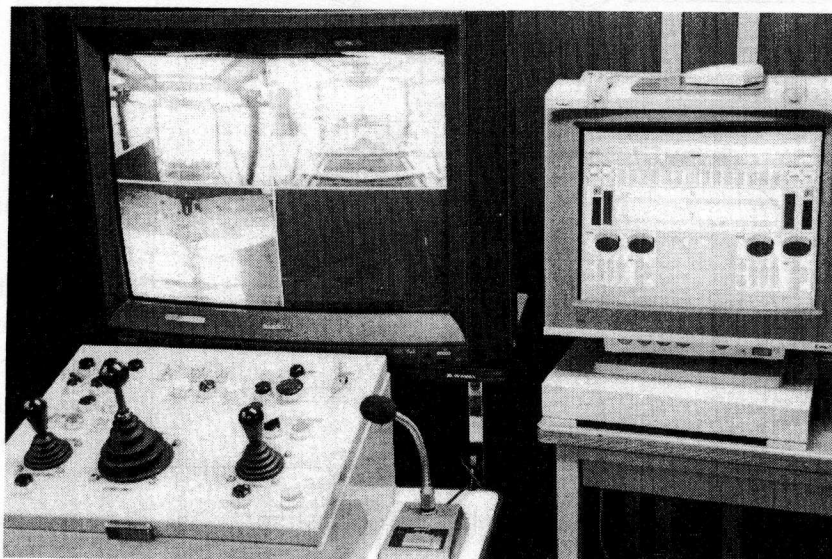
Photo 1. Central control unit
