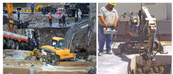
c. Restoration work in condition with out-of-sight
