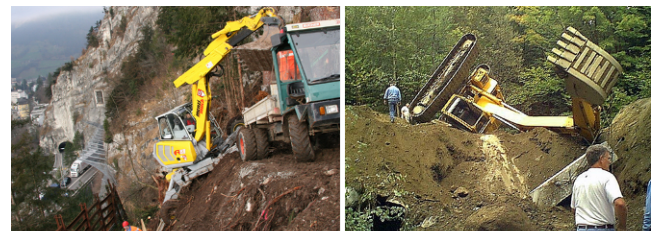
a. Earthwork in slope
