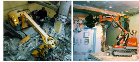
b. Remote controlled demolisher - Brokk100 (BROKK, UK)
