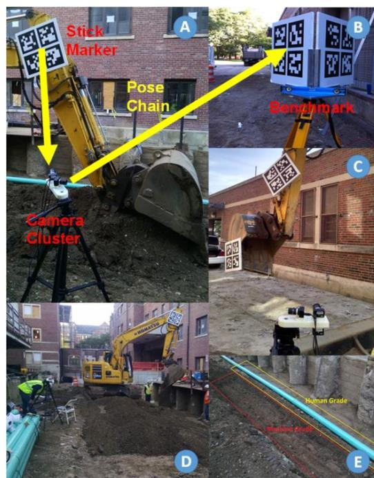
Figure 1. SmartDig: (A) camera cluster and stick marker; (B) benchmark with pre-surveyed pose in the project reference frame; (C) system calibration; (D) working prototype of automatic grade control; (E) comparison to manual grade
