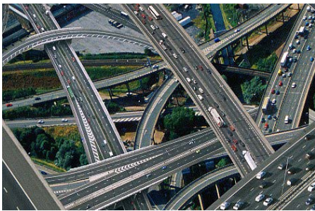
Figure 2- Flyover bridges “Spaghetti”
