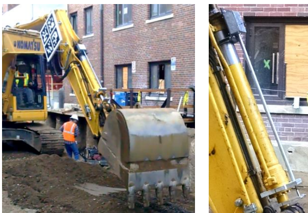
Figure 17. Cable potentiometer site testing
