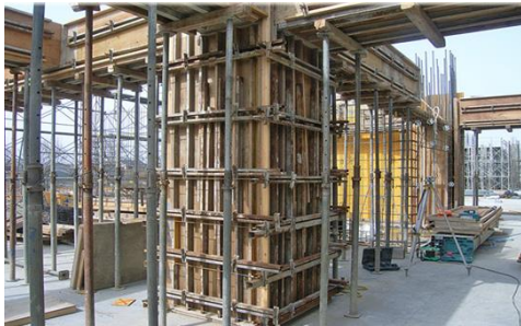
Figure 2. Conventional column and beam formwork[10]
