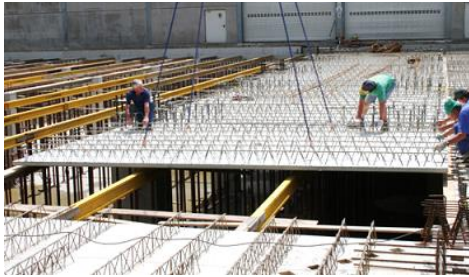
Figure 1. L method (Cast in lattice girders PC slab)[9]
