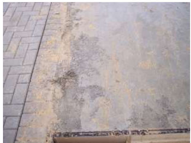
Fig. 3. Frost destruction of the concrete slab surface at the gas station
