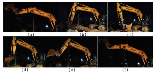
Figure 20. Experiment order of digging work
