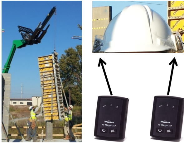
Figure 1. Activity monitoring “stripping formwork off concrete columns” with GPS data loggers on workers’ hardhats
