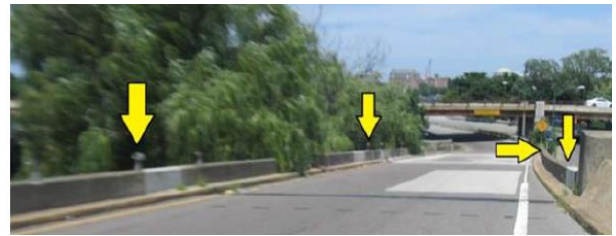
Figure 1. Missing railings from the bridge, however, drawings do not reflect the situation on the ground
