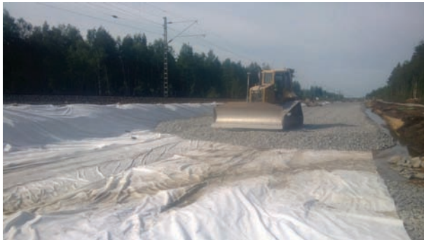
Fig. 1. Photo from Riippa-Eskola railway construction project.
