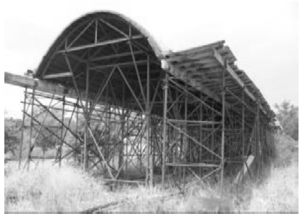
Fig.1. Construction of a ceramic surface by Eladio Dieste using extensive scaffolding, (Image courtesy of Prof. Martin Bechthold)
