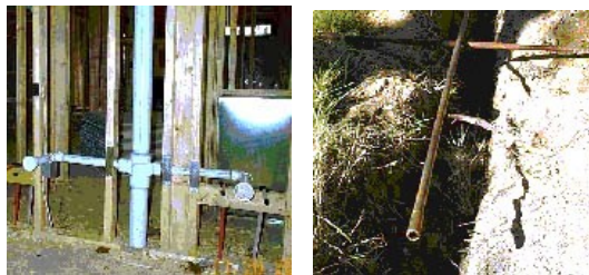
a) Studs, Plumbing, Power b) Buried Water Line
