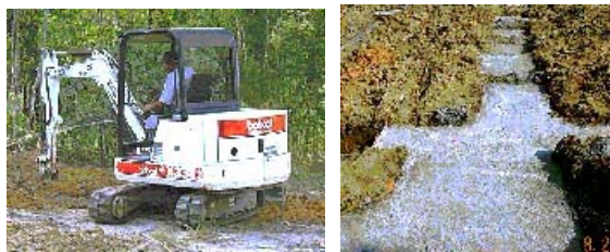
Fig 6. Remote Inspection of Foundation Using SWS
