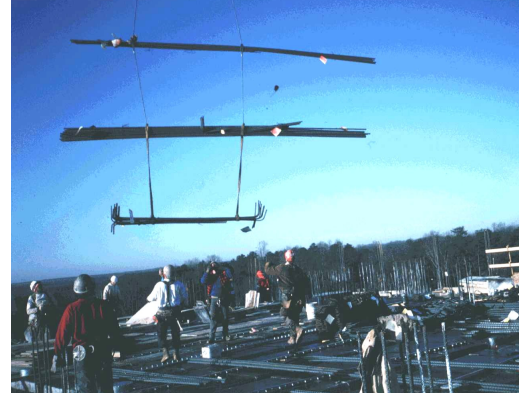
Fig 2. Rebar delivered according to the sequence of placement
