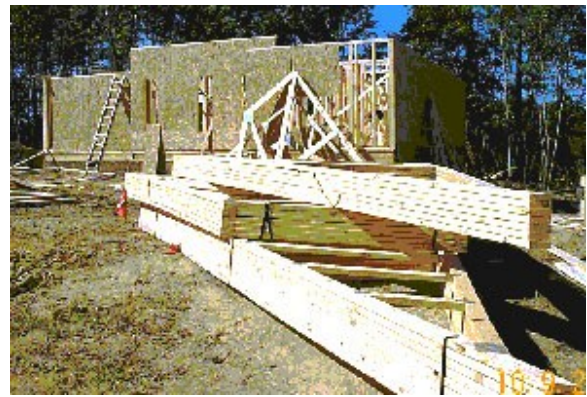
b) Wall Framing is Being Worked on, Roof Trusses Are Delivered
