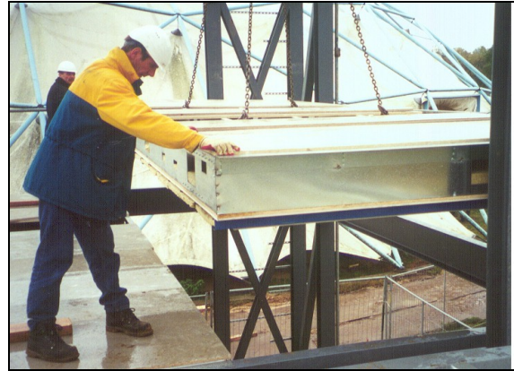
Figure 2. Assembling the floor panels.
