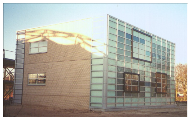
Figure 3. IFD building system trial module on the Eindhoven University of Technology campus.
