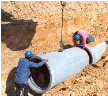
a) Laying Pipe Traditionally
