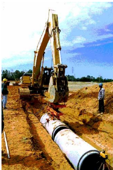
b) Laying Pipe with PipeMan c)
