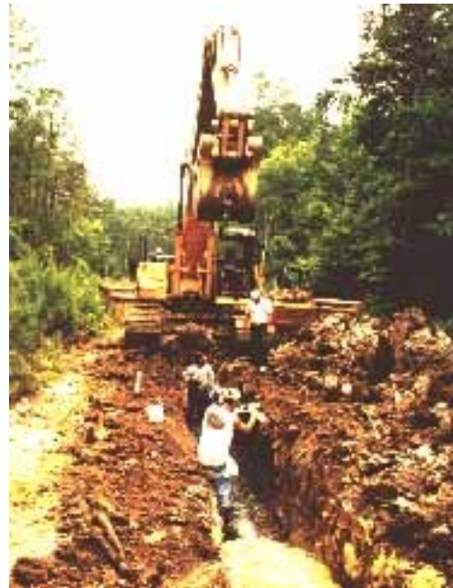
Fig 1. Dangerous Work Laying Pipes in an Open Trench
