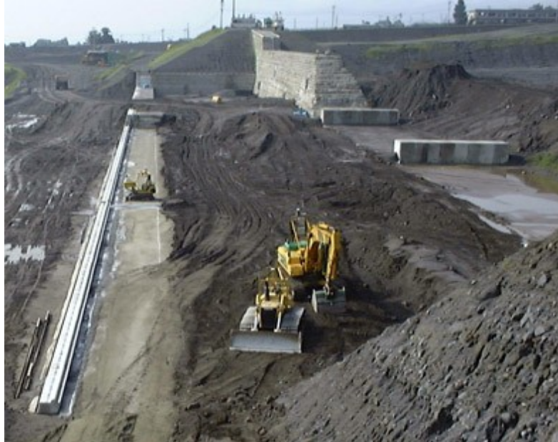
Figure 2: Fujita Tele-Earthwork System in Operation
