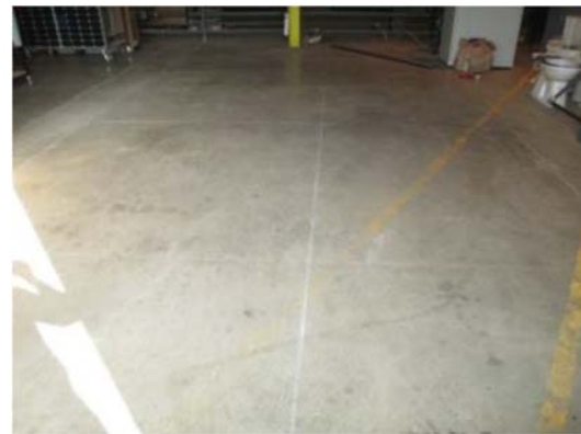
Figure 7. Drainage Lab slab studied in this work.
