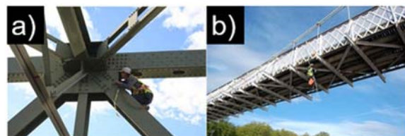
Figure 1. Dangerous bridge inspection (source: icaeng.com, hireuavpro.com).
