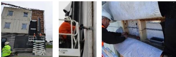
Figure 4. Left: Installing the panels. Middle: Fixing the connector to the wall. Right: Joining
