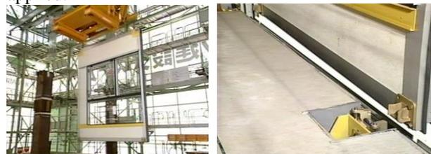
Figure 1. Ideal robotic façade installation by Obayashi. Right: Positioning of the façade element. Left: Compliant plug-and-play connector façade element. (images: Obayashi documentary video) [1].
