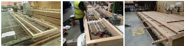
Figure 3: Manufacturing process of the modules. Left: Timber-frame manufacturing. Middle: assembly of services onto the module. Right: Manufacture of finishing grid.
