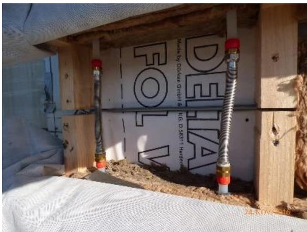
Figure 6. The connecting system with inaccuracies that can be detected even visually.
