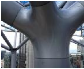
Figure 2. Bevis Marks Roof (Cladding) [28]
