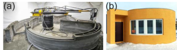
Figure 9. On-site’ 3D printed house by Apis Core (a): Construction using a ‘mobile’ 3D concrete printer, (b): House exterior [19]
