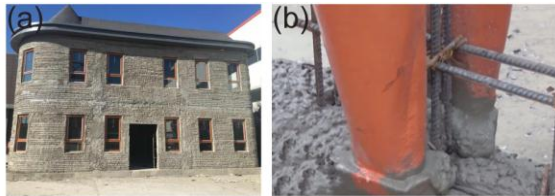
Figure 6. (a): The two-story villa printed by Huashang Tengda company and (b): the novel nozzle of the giant 3D printer [16]
