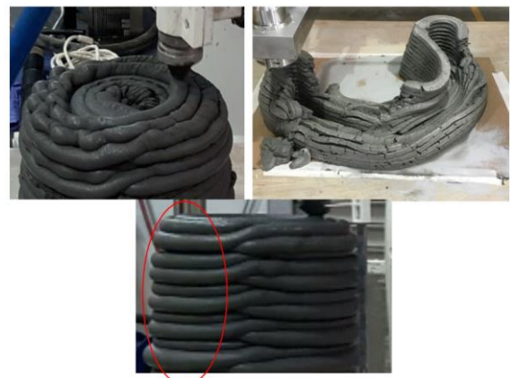
Figure 4. Failures in concrete printing
