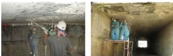
Figure 1 Chipping process by manpower
