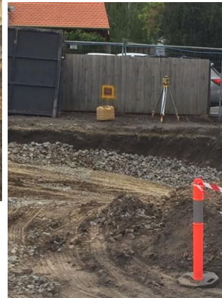
Figure 6. TopCon Laser transmitter with string line in view
