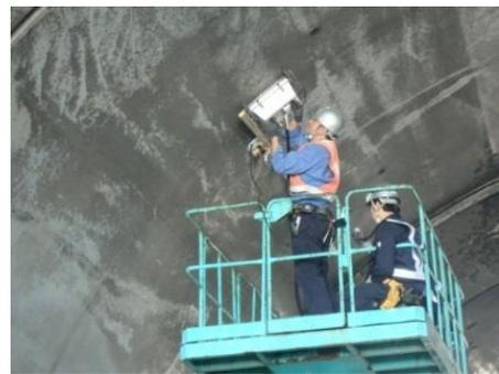
Figure 8. Tunnel inspection by using our device on an aerial work platform
