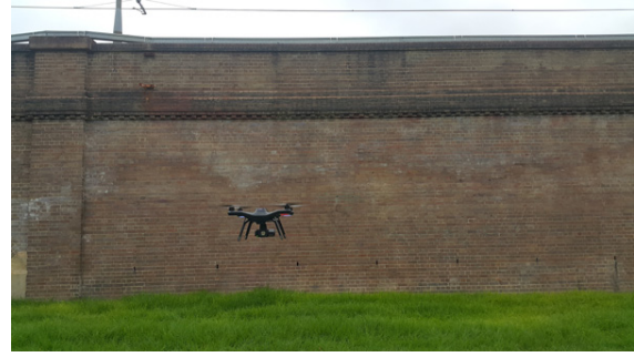
Figure 3: Collecting data of the bridge.
