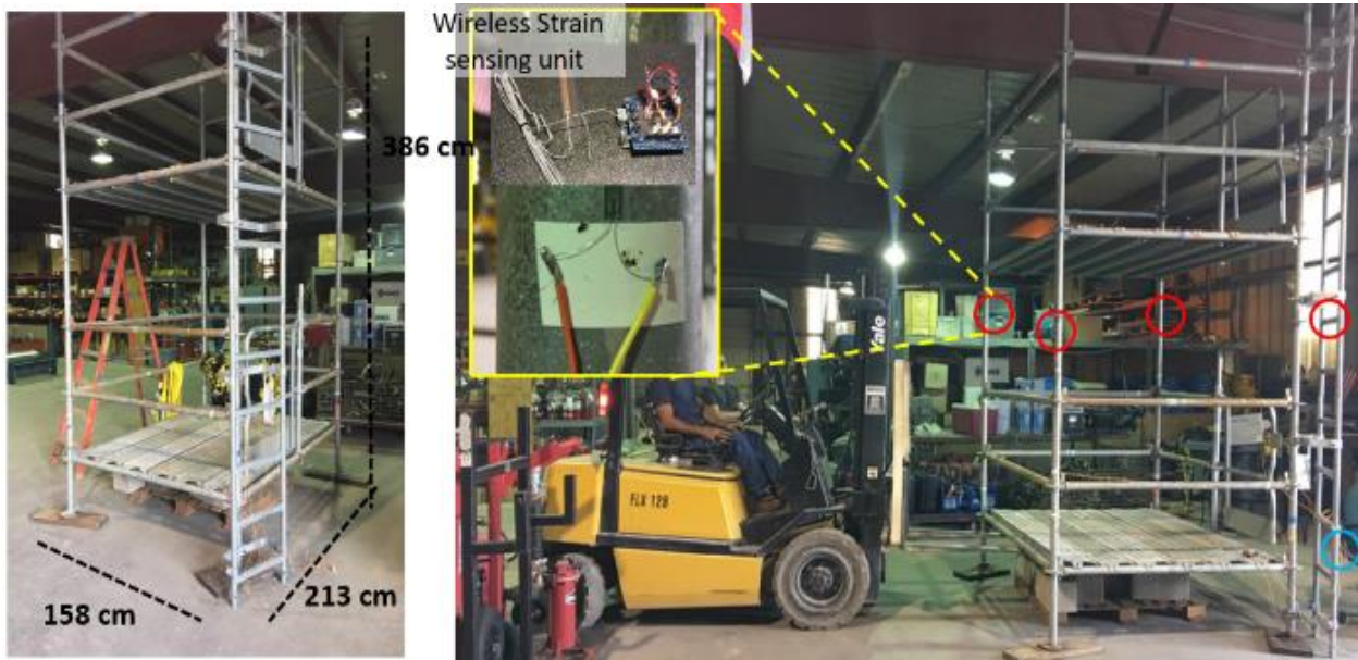
Figure 4 Experimental setup with a one-bay scaffold
