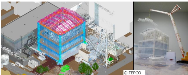
Figure 3. Temporary Cover over the Damaged Reactor Building of Unit 1
