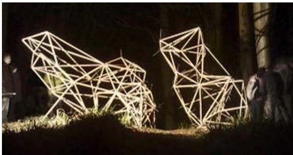
Figure 3 and 4. Human collaborators installing timber elements guided by the cable robot pointer, resulting in a variable density triangulated structure
