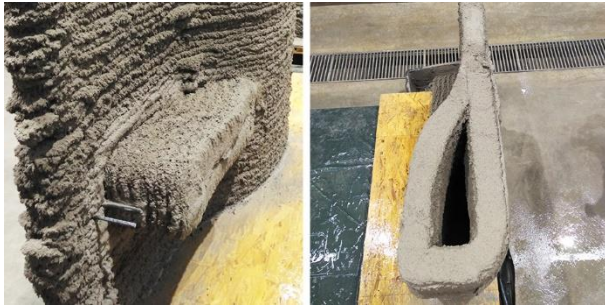
Figure 11. Wall produced with Shotcrete 3D Printing; Detail of the console, with 2 reinforcement bars left blank (left); top view of the wall (right)
