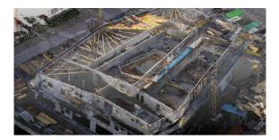
Figure 2. Occluded construction elements in generated point cloud caused by scaffolding, formworks, existing elements and missing information during the reconstruction process
