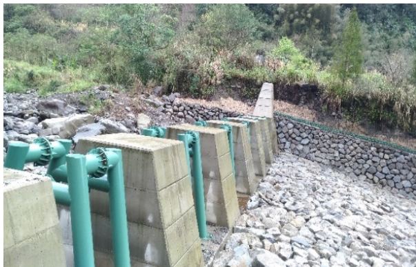
Figure 7. Steel-pipe-type slit dam of the case project
