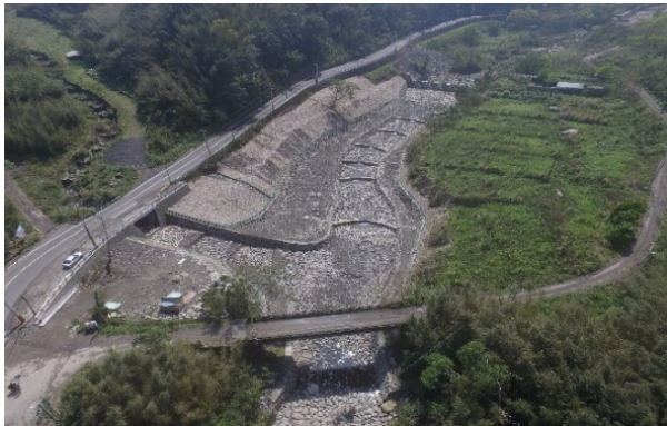
Figure 6. Bird's view of case project
