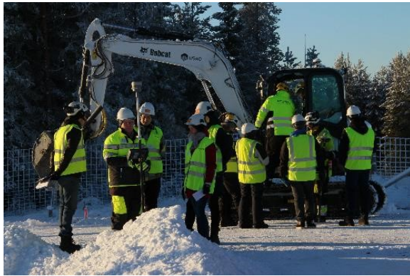
Figure 6. Trimble R10-RTK-GNSS-system (trick 6) and Bobcat excavator with both 3D-guidance systems of Scanlaser and Novatron (trick 5).
