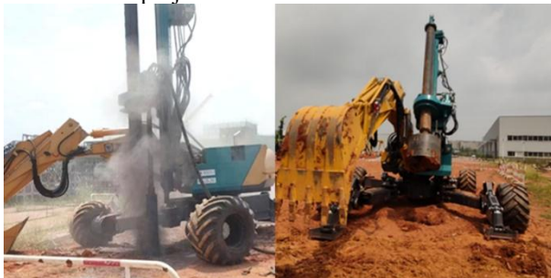
Figure 3. Real-World Drilling and Excavation Scene of the Mechanized Platform
