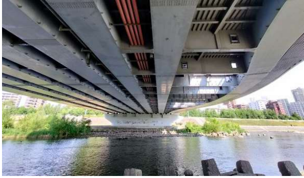
Figure 2. An example of the underside of a bridge
