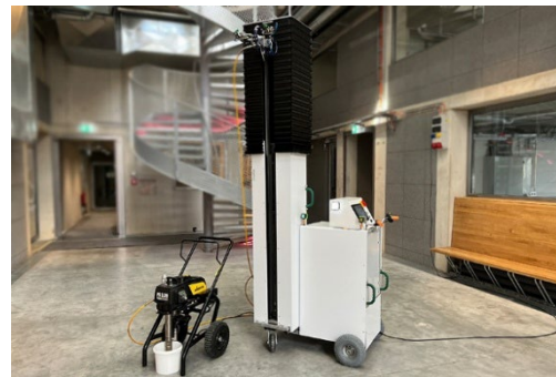
Figure 2. Nova-S spraying modular robot with dual nozzle. The external pump attached to the robot ensures material flow. [18]
